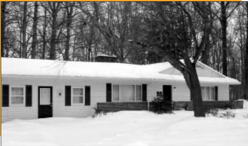
AWP's new office building, Carty House after a snow storm this past winter.
